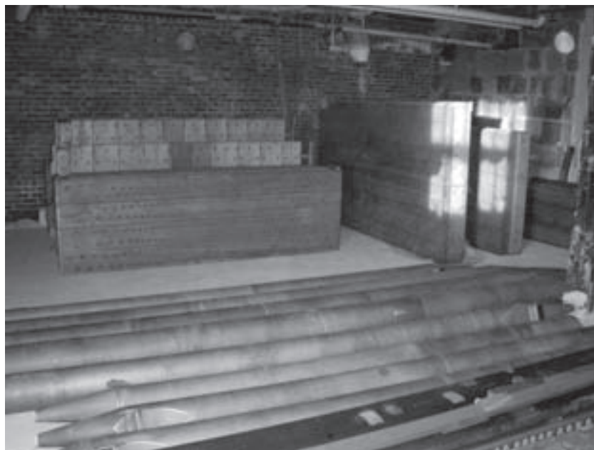
The Left Stage chamber has had all the windchests for the Swell Organ removed to be sent out for restoration. The top photo shows the vertical void created by the chest removal and the lower photo shows the windchests stacked up in a secure room awaiting shipment.
