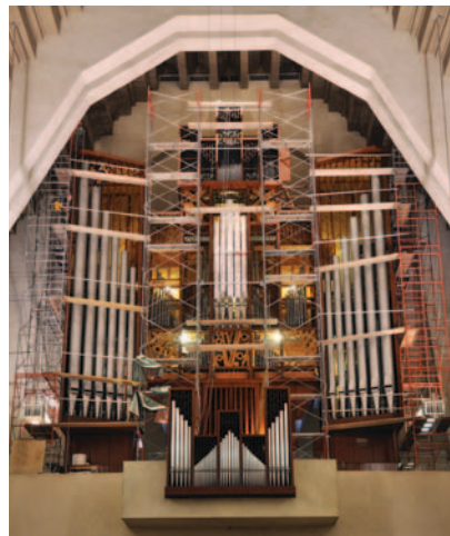
The case covered in scaffold (photo credit: Robin Côté)
