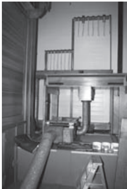
Pedal organ chassis being reinstalled
