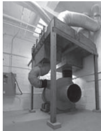
The restored Spencer blower for the ballroom Kimball organ
