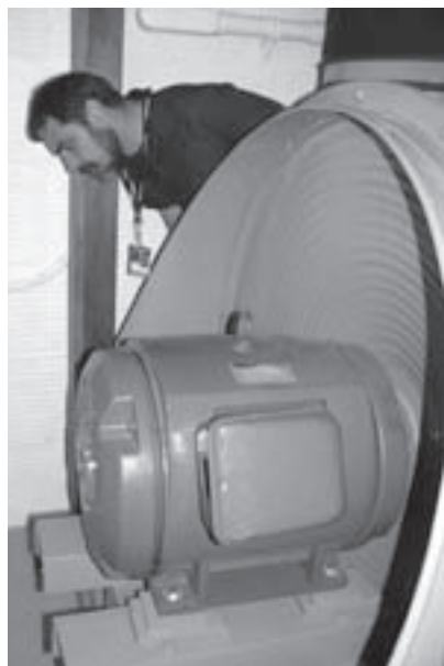
View of the restored blower motor for the ballroom Kimball organ. Curator Carl Loeser looks on.
