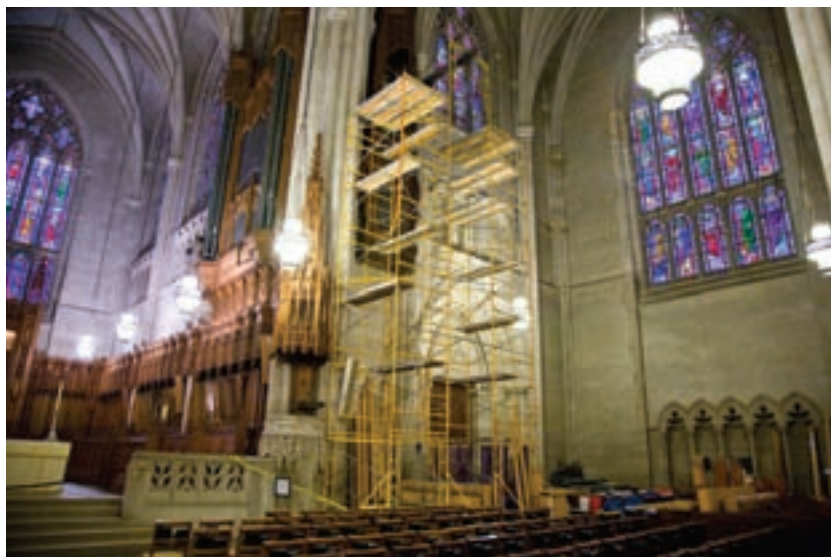
Scaffolding was 50 feet high to remove Great/Pedal/Choir/Swell equipment
