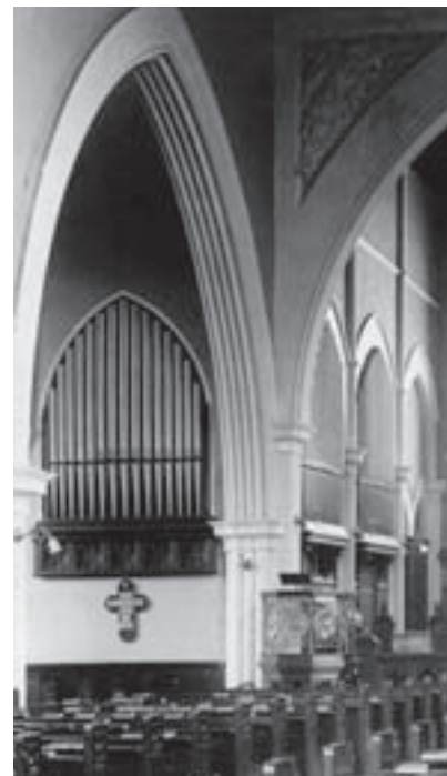
Original 1902 Kimball façade
