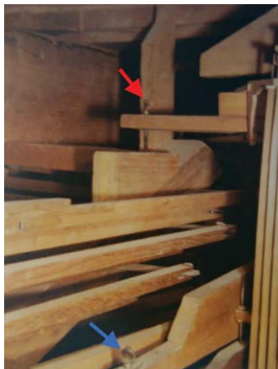
Looking from the front of the console to the left of the keyboards, we see a blue arrow pointing to the adjustment screw for the Swell action and a red arrow pointing to the adjustment screw for the square rail of the Great action, which is fanned (notice the angle of the square).
