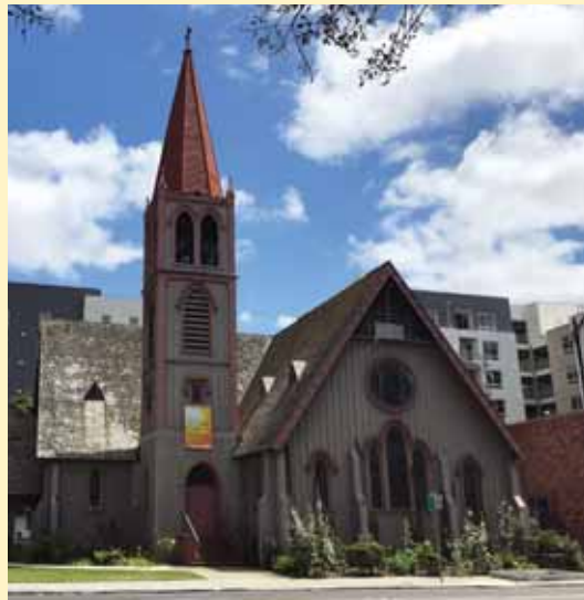
Trinity Episcopal Cathedral, San Jose, California (photo credit: Paul Archambeault)
