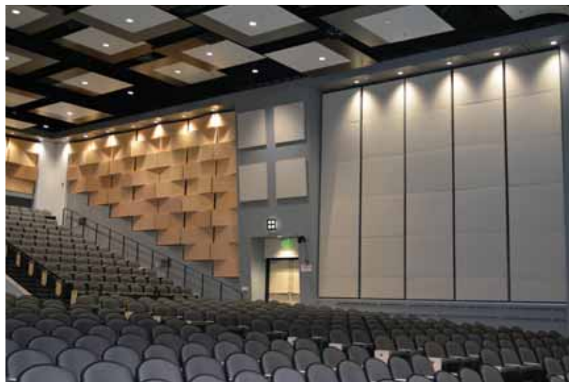
Shari Fleming Center for the Arts, sound reflective and diffusing wall panels revealed at side/rear wall near elevated seating, with sound absorbing wall panels revealed at forward taller side wall (photo credit: Richard Lenz)
