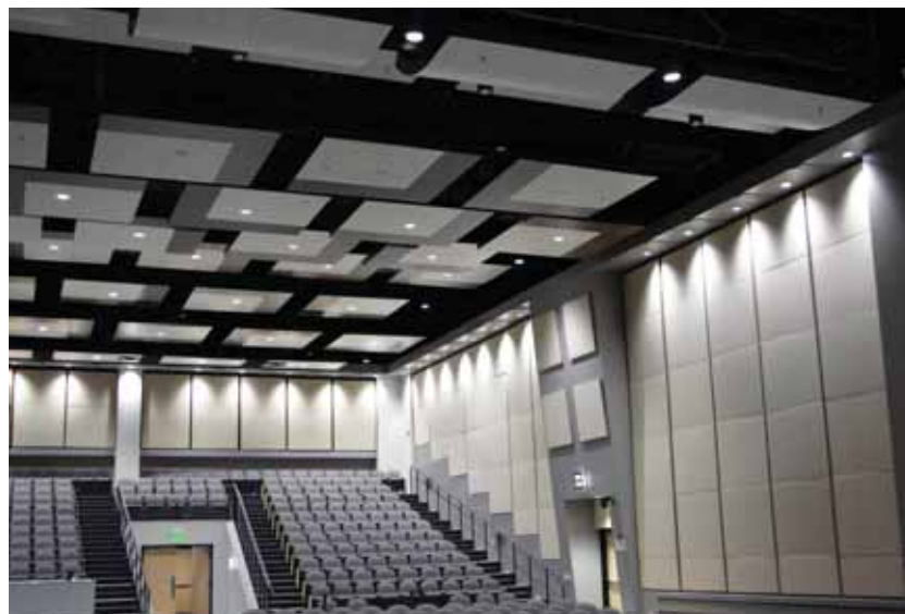
Shari Fleming Center for the Arts, Tabor College, Hillsboro, Kansas, sound absorbing wall panels revealed at all side and rear walls (photo credit: Richard Lenz)
