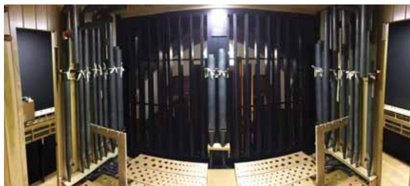
Reinstallation of the organ has begun. (photo credit: Berghaus Organ Company)
