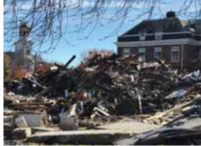
First Baptist Church, Wakefield, Massachusetts, after the fire of October 23, 2018 (photo credit: John Boody)
