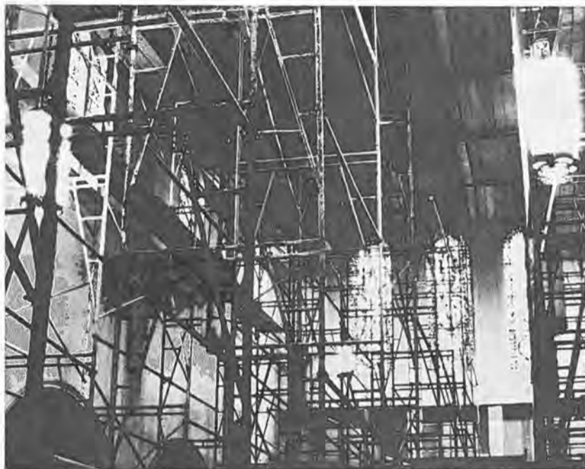
View of acoustical renovation in progress at All Saints' Church
