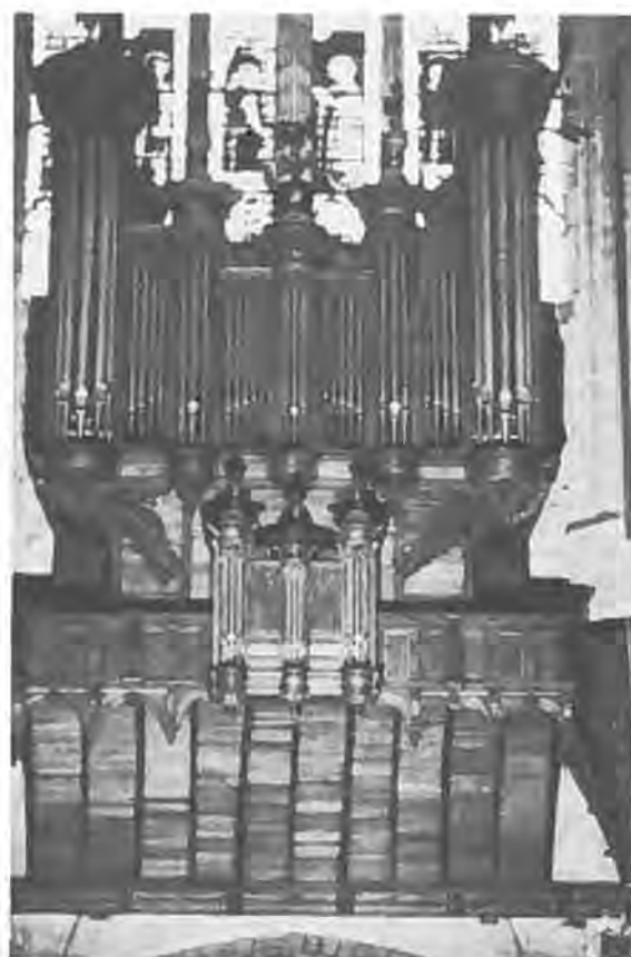
Bourges Cathedral, France. Total restoration by Kern of Strasbourg in 1985 included attached console, mechanical stop action and 3 ventii pedals as the only registration aids.
