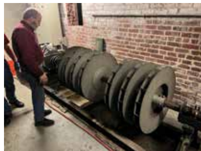
Curt Mangel inspects the fan assembly of the high-pressure Swell division (100 horsepower, 1750 rpm, eighty-inch static wind pressure) of the Boardwalk Hall organ, Atlantic City, New Jersey. Notice the bearings in oil bath at far right. (photo credit: Carl Hersom)
