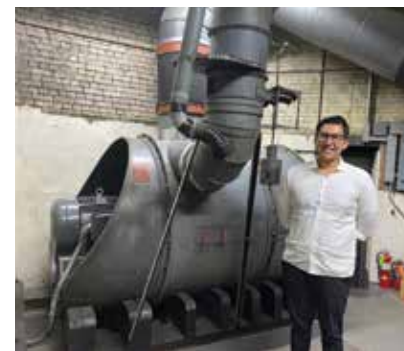
Former associate organist Michael Hey (well over six feet tall) and the forty-horsepower blower of the Kilgen organ at Saint Patrick's Cathedral, New York, New York (photo credit: John Bishop)
