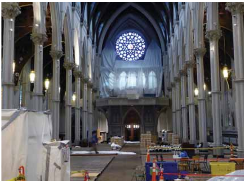
Holy Cross Cathedral, Boston (1875 E. & G. G. Hook & Hastings Opus 801), partial dismantling to protect the organ during building renovation. Project by Andover Organ Company and the Organ Clearing House. (photo credit: Matthew Bellocchio)
