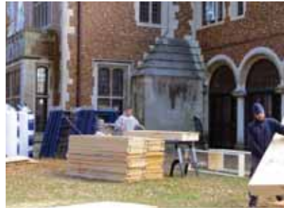
Building pipe trays. "Tubes" containing three rolls of styrofoam are visible in back left. (photo credit: John Bishop)
