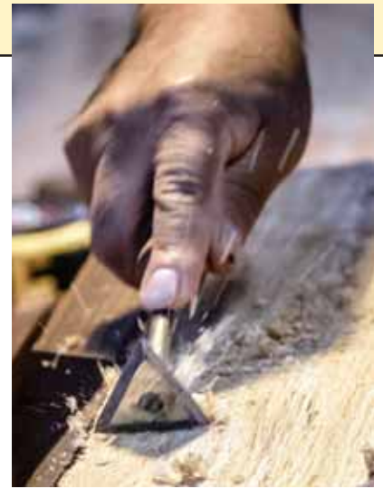
Preparing wood surface with a scraping tool (Peragallo)
