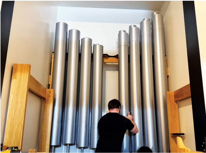
Choir 16' pipes being installed
