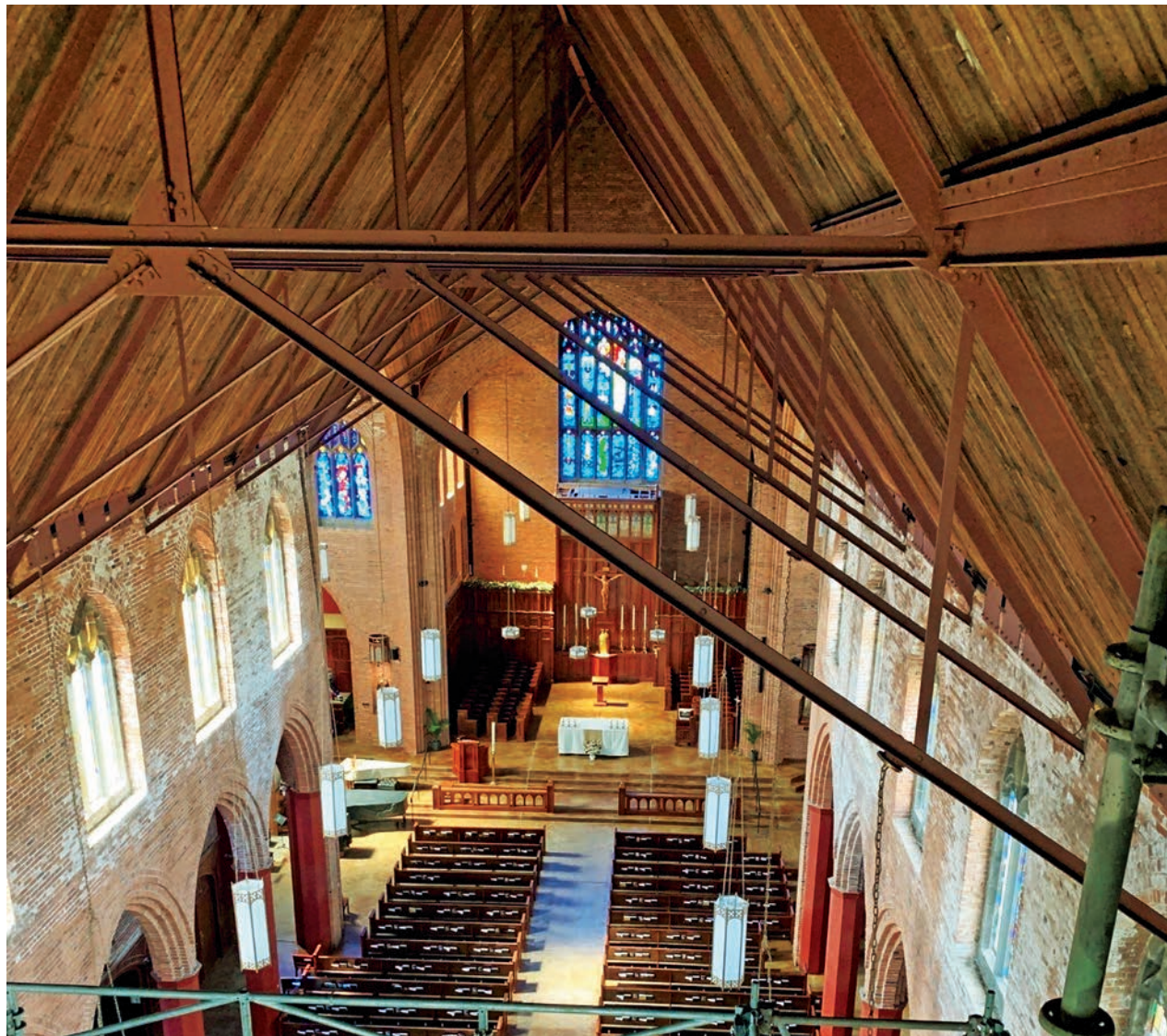
View from the top of the 68-foot-tall scaffolding erected with two hoists, one to lift parts to the level of the 35-foot-high loft and one to lift them as high as the top of the Swell division 26 feet above the loft floor.
