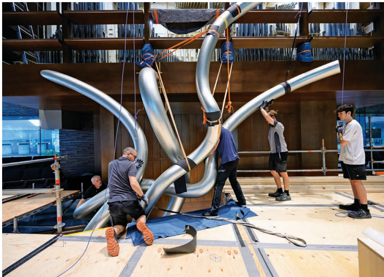
During the assembly of the sculptural façade pipes, which serve as a 16' Violonbass and wind channel
