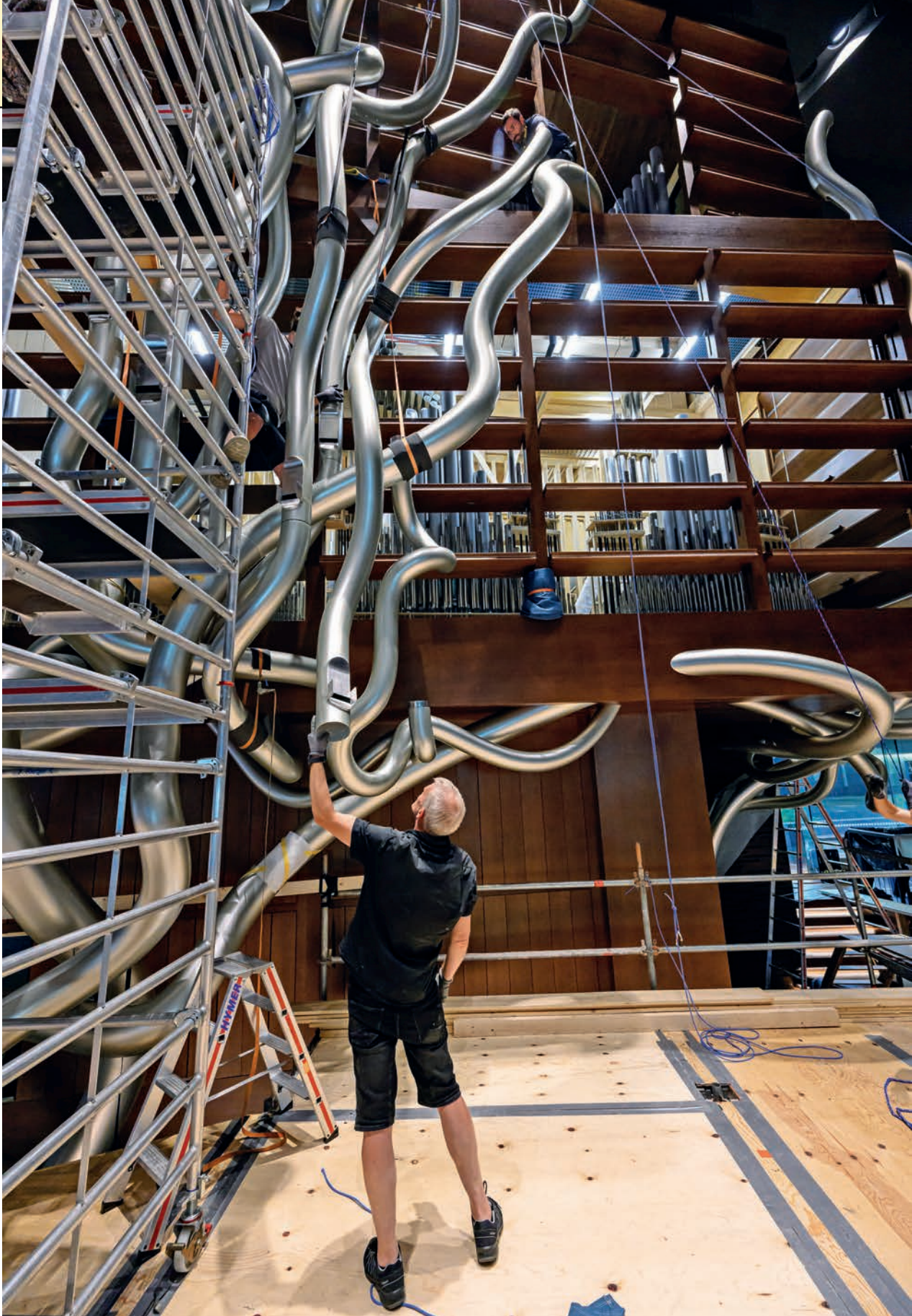
Installation of the individual façade pipes
