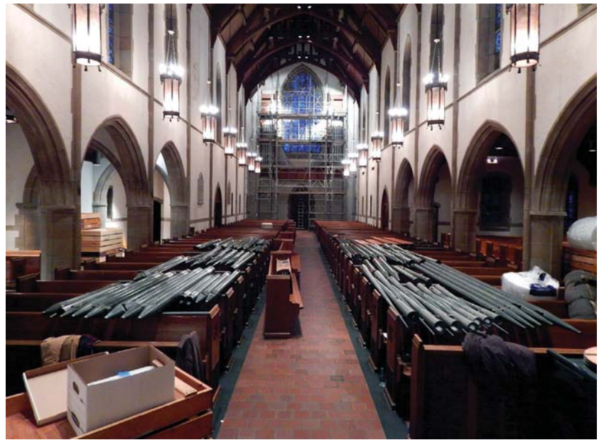
Removal of pipework
