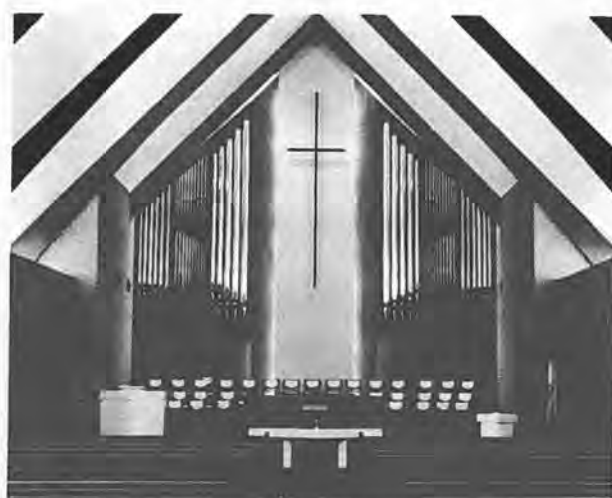
FIRST PRESBYTERIAN CHURCH OF MAITLAND, MAITLAND, FLORIDA
