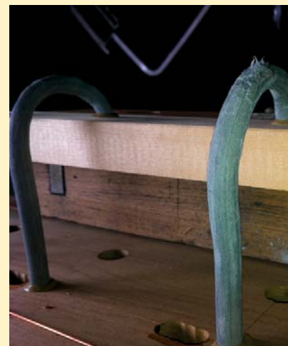
Lead tubing, before
