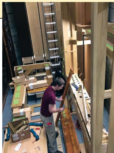
Ryan Mueller installing Pedal bass chests
