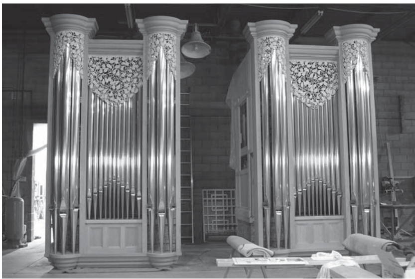
Gallery rail cases under construction
