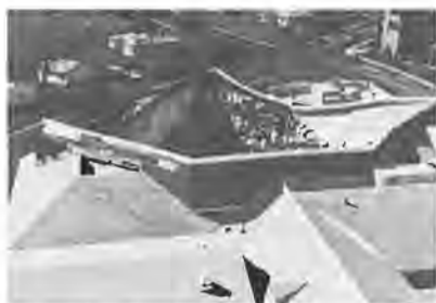
View of auditorium roof
