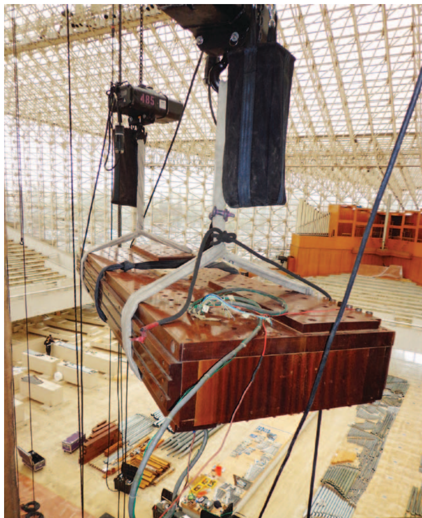
Ruffatti windchests being lowered to floor level
