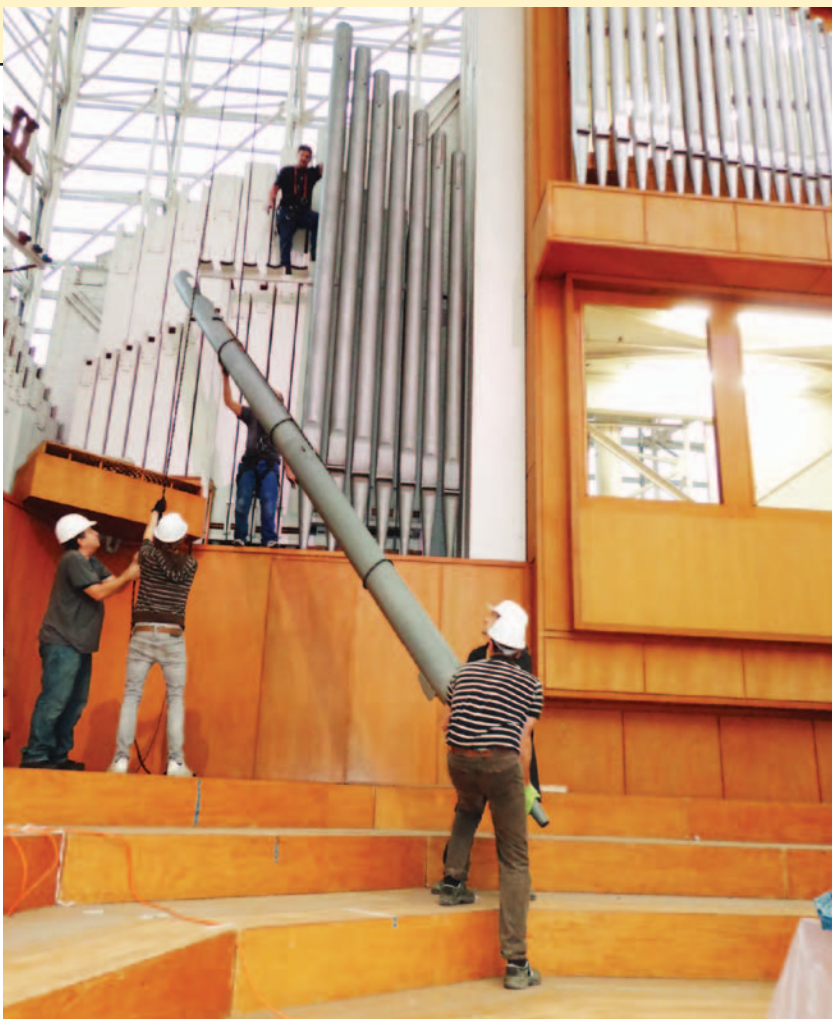
Front organ: large façade pipes being removed
