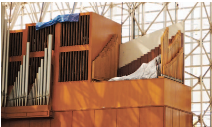
Gallery organ, prior to restoration. Several areas of the organ were temporarily protected to limit the damage from rainwater from leaks in the roof.
