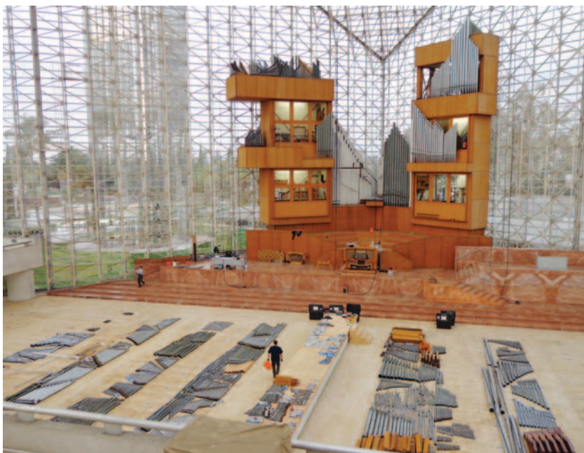
The organ's disassembly: all chairs have been removed from the cathedral floor and pipes are being carefully stored over the entire floor area, waiting to be packed.
