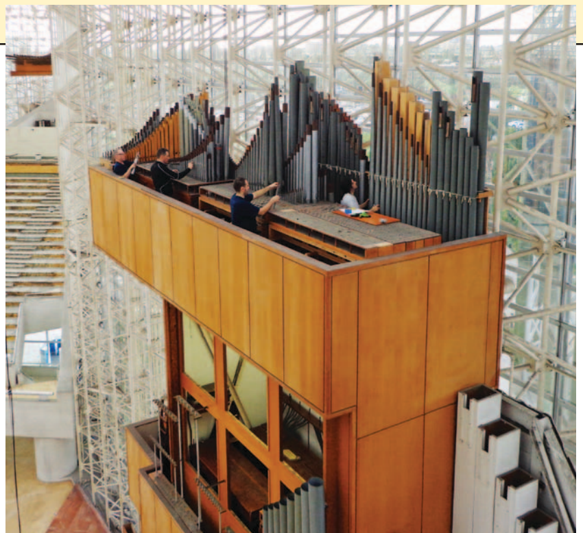
Pipes being removed from the highest level of the front organ
