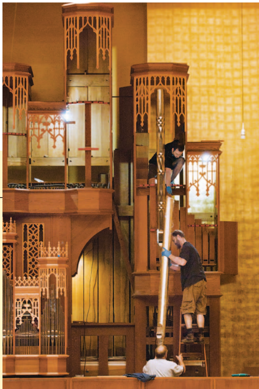
Installation of the façade pipes (photo credit: Kathleen Karn, UC Berkeley)
