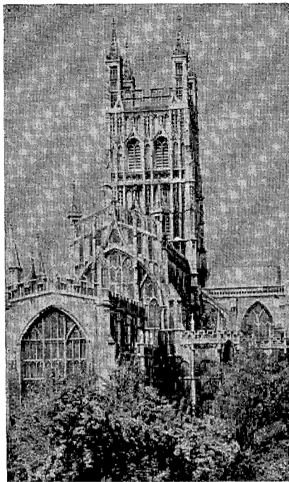
Great tower of Gloucester Cathedral completed about 1450 is said to weigh about 4700 tons.
