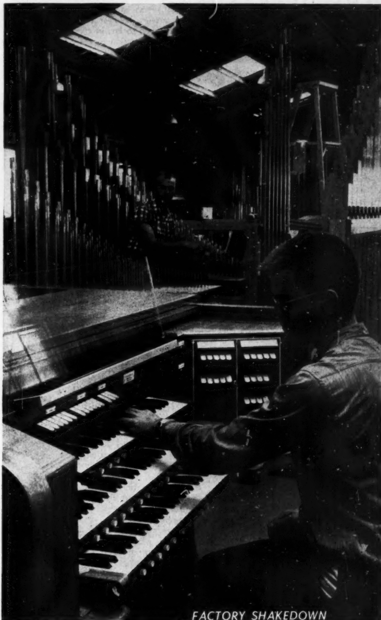
An organ built over a period of about 10 months for a church in Louisiana gets a final shakedown, with pipes exposed, in the plant before being shipped. Harrison Heth, a trained organist whose job at the factory is voicing pipes, is at the console of three manuals, or rows of keys. Listening is Don Johnson of Chicago, who is taking installation training at the factory.
