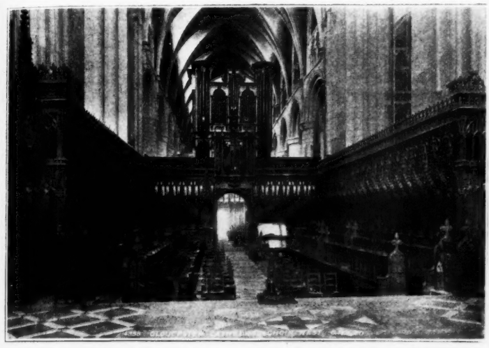
VIEW OF GLOUCESTER CATHEDRAL SHOWING ORGAN.
