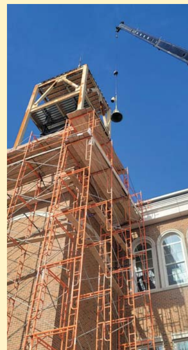
Hoisting a bell into the tower
