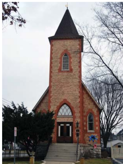
The original Grace Lutheran Church
