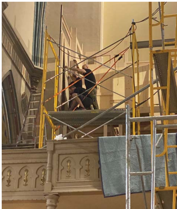
Amory Atkins, Joshua Wood, and Terence Atkin of the Organ Clearing House assembling the Swell box of Noack Opus 164, Cathedral of Saint Paul, Birmingham, Alabama (photo credit: John Bishop)
