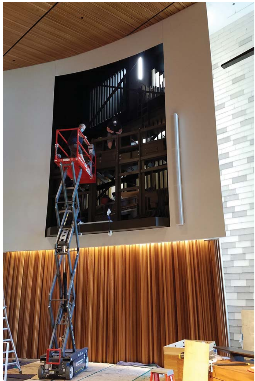
A scissors-lift replaces scaffolding
