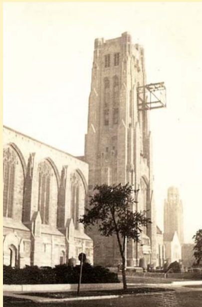
Installation of bells in progress in 1932
