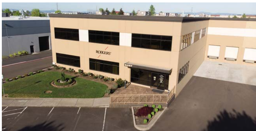
Rodgers Instruments US, LLC, new facility
