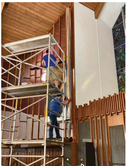
First façade pipe being installed
