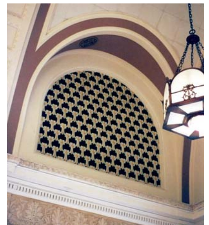
One of the tonal openings for the original 1930 Geo. Kilgen & Sons Opus 4524
