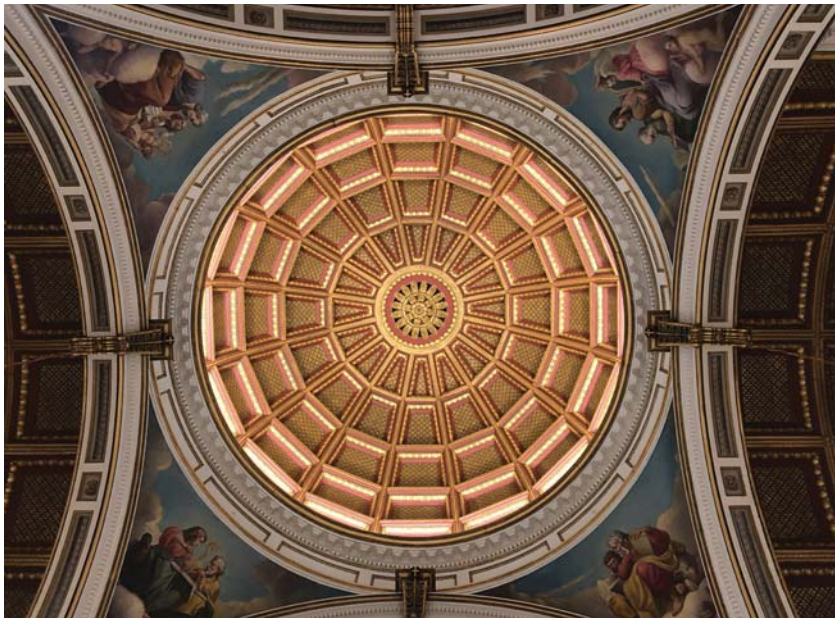
Dome above nave crossing
