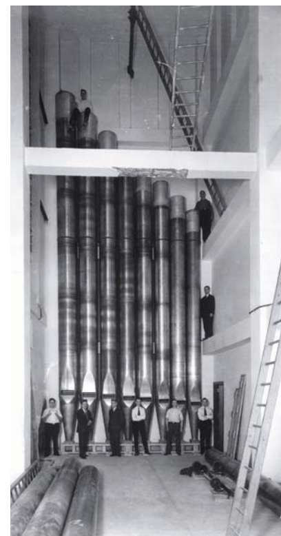
There are ten 32’ stops in the organ, including the Pedal-Left Diapason seen here. The 32’ pipe (at left) has a diameter of 24 inches and is thought to be the world’s heaviest metal organ pipe—2,200 pounds. It is made from 5/16” thick zinc that was cold-rolled on a machine designed for making ocean liner funnels.
