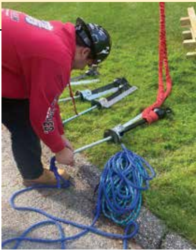
Jake from the Verdin Company preparing bell strikers for hoisting (photo credit: John Bishop)
