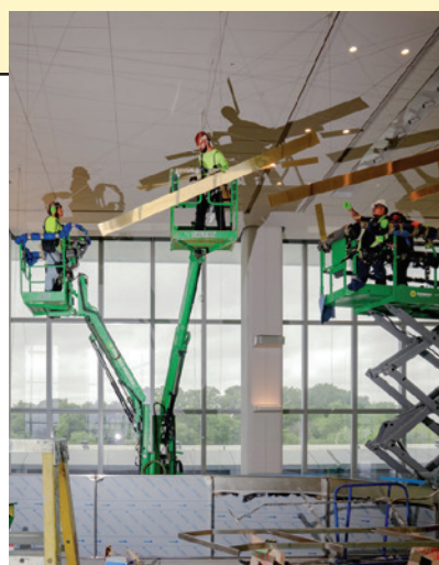
Orpheus and Apollo during its installation in LaGuardia Airport. The crew had to reassemble 188 metal bars, suspended at precise angles midair, from 444 wires attached to the ceiling. (photo credit: AMIR HAMJA/The New York Times/Redux)
