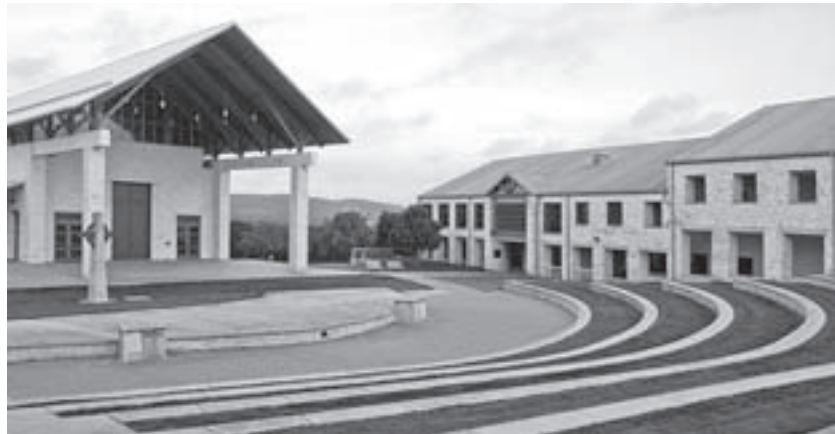
Architect Chris Carson’s new TMI Chapel is the focal point of the campus, located in the rolling hills of northern San Antonio.
