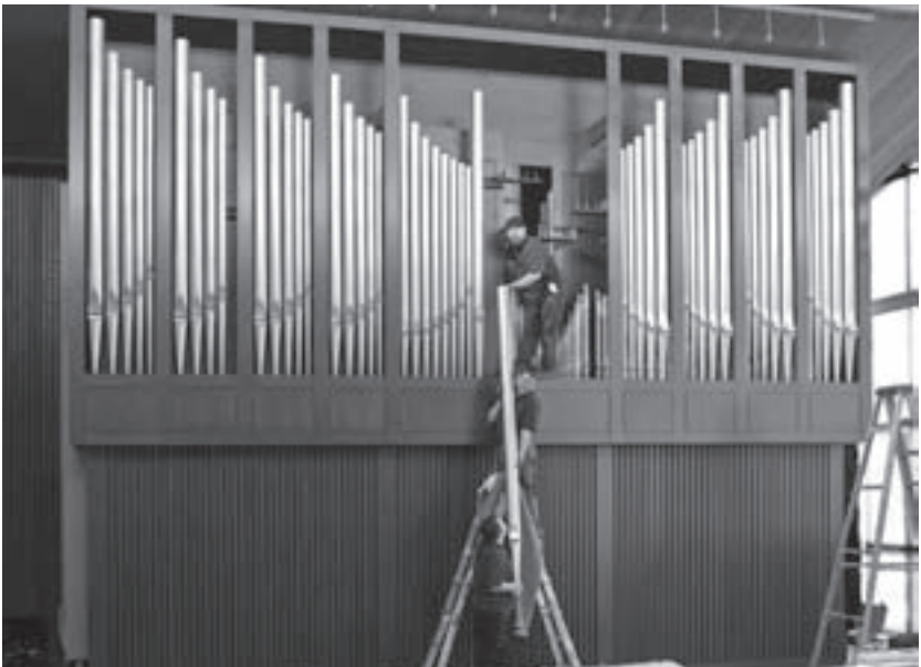
Day 7: The display, utilizing pipes from the Open Diapason, Harmonic Flute and Pedal Principal, brings the organ closer to completion. After tonal finishing, the organ will be used for chapel services as well as diocesan events, all under the leadership of the school's music director, Dr. Thomas Lee.
