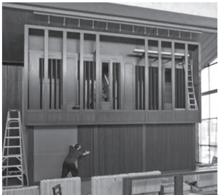
Day 5: The lower case nears completion. Other detail work continues inside the organ, such as connecting chest cables to the relay and winding details.
