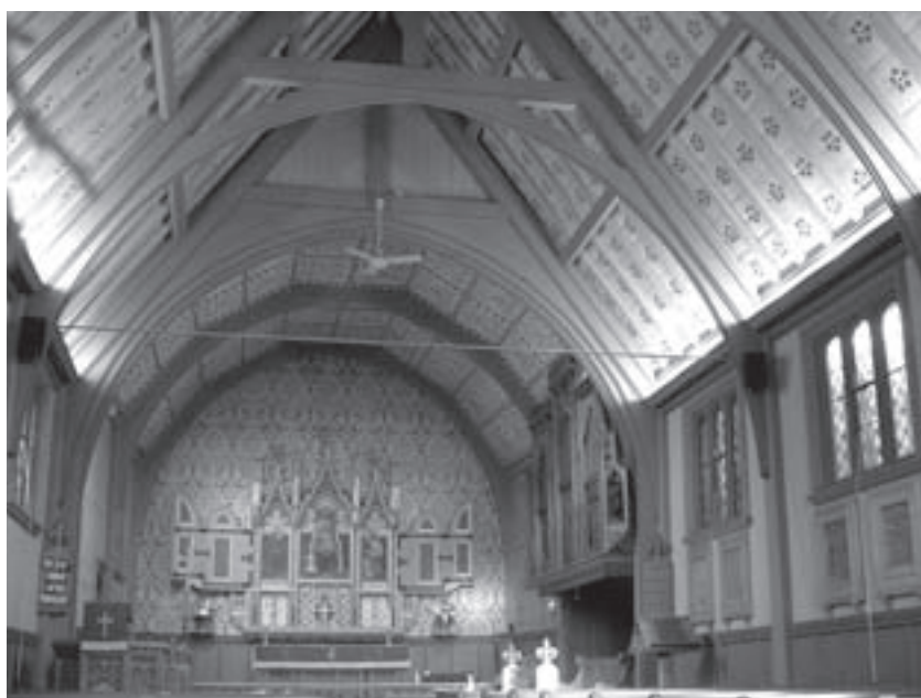
Church interior (photo credit: Jay Zoller)
