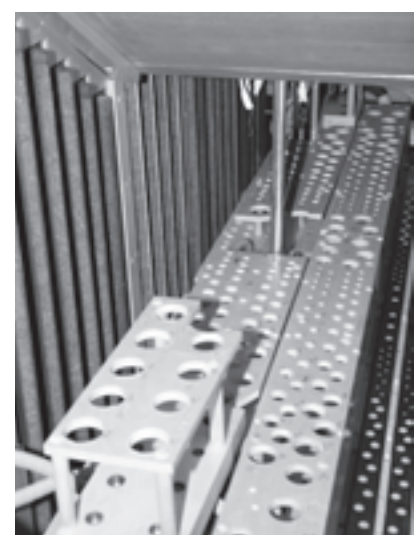
The interior of the Rückpositiv is ready for pipe installation (photo credit: Ron Turner)
