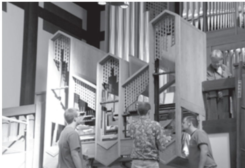
Roy Redman oversees installation of Rückpositiv casework (photo credit: Ron Turner)
