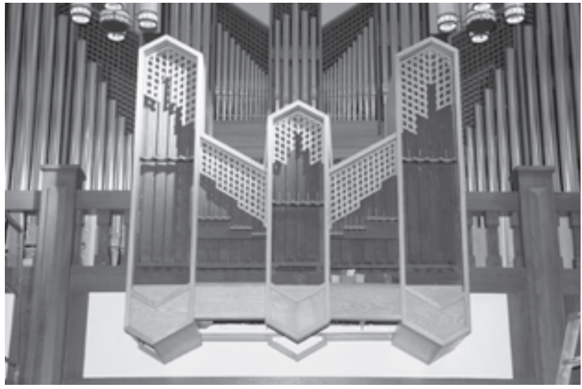
Rückpositiv casework is in place and ready for installation of façade pipes (photo credit: Ron Turner)
