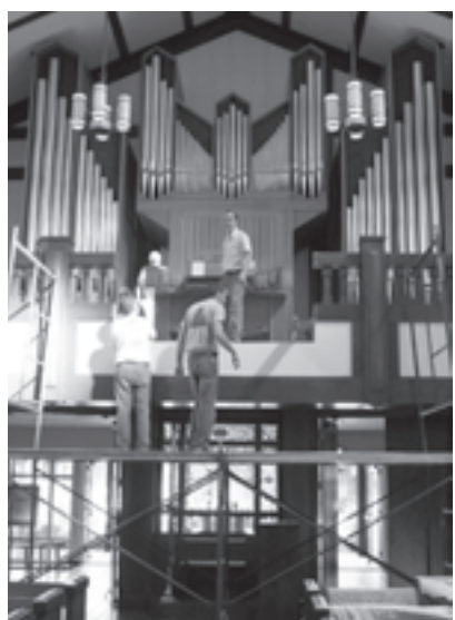
Installation of steel beams to support new Rückpositiv (photo credit: Ron Turner)
