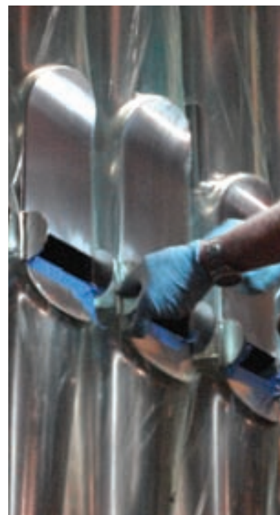
Adjusting façade pipes (photo: Margaret Gettig)
