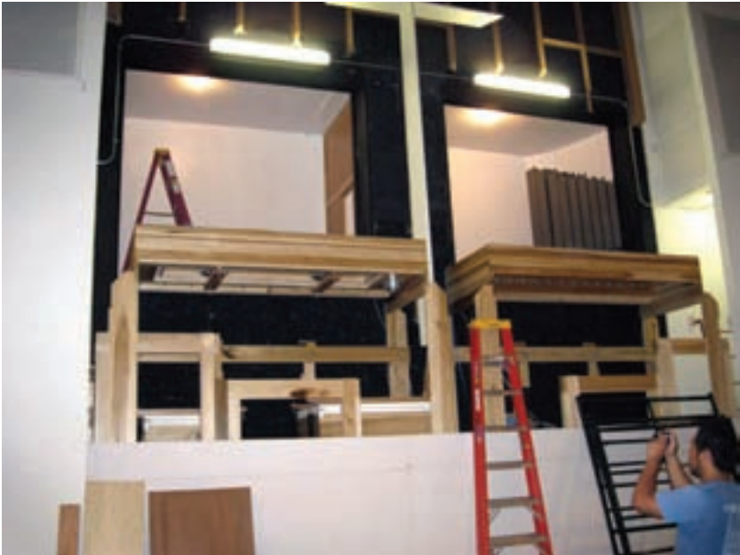
Great slider windchests being installed
