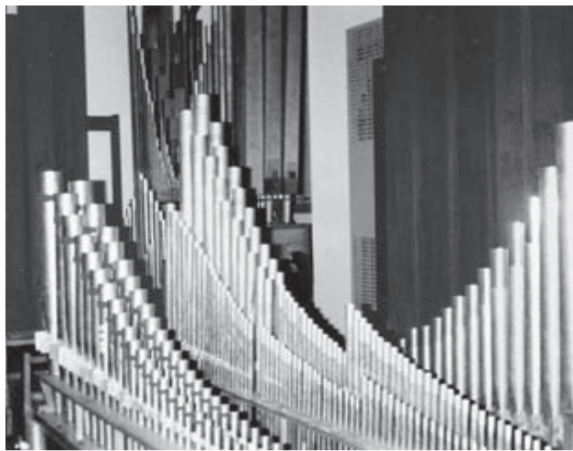
Organ installed in Hinsdale house in 1977
