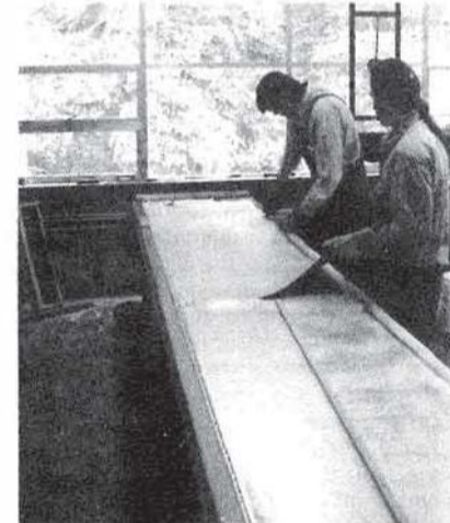
6) Pipe metal hardens almost immediately.
