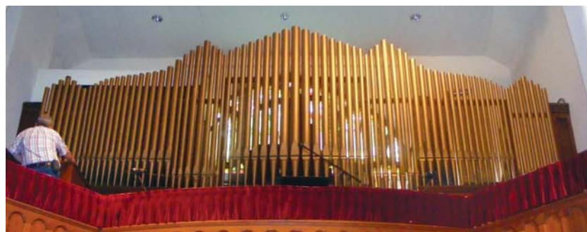
Examining the façade pipes
