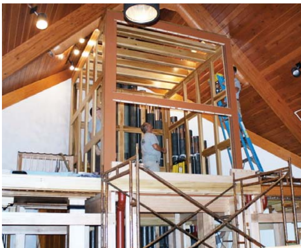
Erecting client-built Swell enclosure (photo credit: Rev. Kirk Clayton, Zion Lutheran Church)
